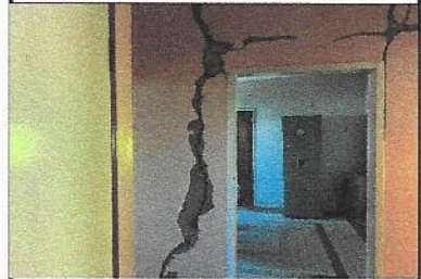
Wall cracks
